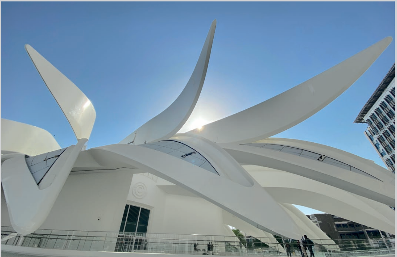
EXPO 2020 Dubai, UAE Hydraulic motion system for controlling the opening and closing of the roof of the UAE Pavilion
